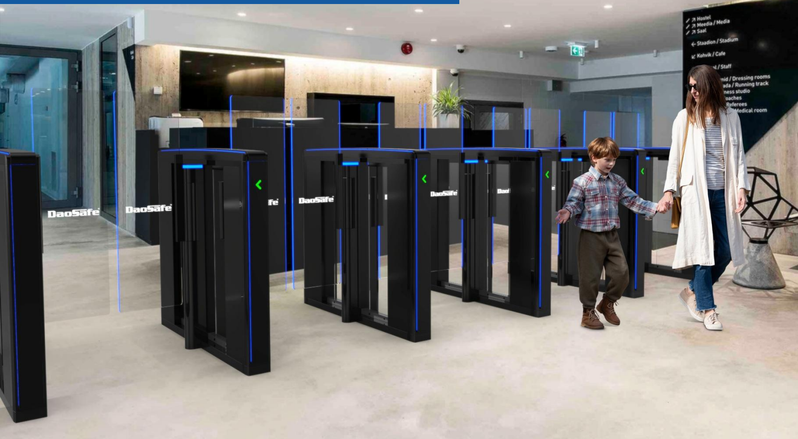
Five lanes high glass installed at media
